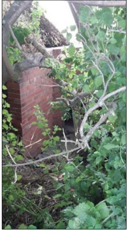
View 4: Brickwork headwall
