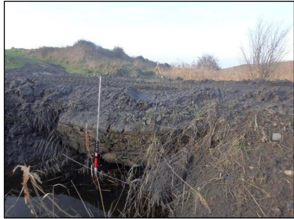
View 2: Upstream view of culvert crossing to the east of the Project road.
