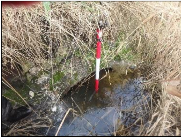
View 3: Upstream view of culvert crossing to the west of the Project road.
