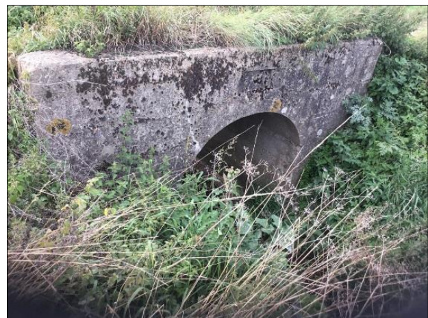
View 6: Golden Bridge Sewer (ref. G)
