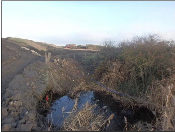
View 1: West Tilbury Main
